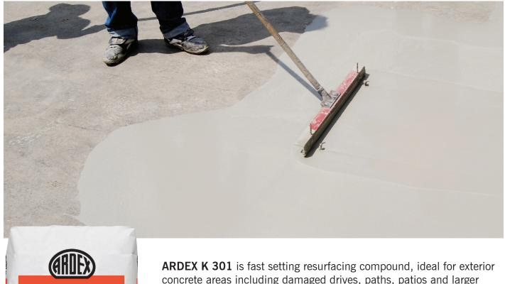
**ARDEX K 301** is fast setting resurfacing compound, ideal for exterior concrete areas including damaged drives, paths, patios and larger surface areas such as domestic car parks and courtyards. It is easy to mix and apply and can be pumped for faster application.
