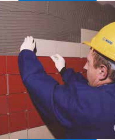
Fixing ceramic tiles on walls working from the top to the bottom
