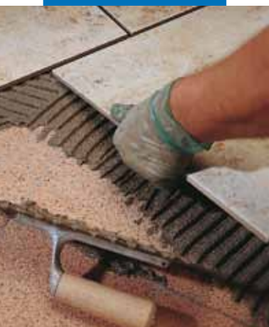
Single-fired tile on terrazzo tile of an external wall
