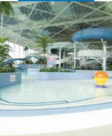
An example of an installation of glazed ceramic pool tiles. Leisure centre
