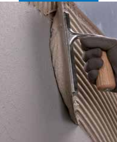
Installing floor covering using Ultramastic III
