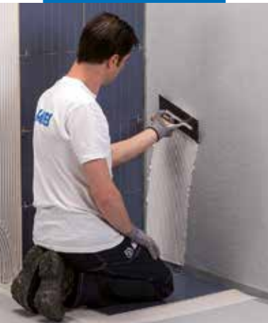
Installing wall covering using Keraflex Maxi S1
