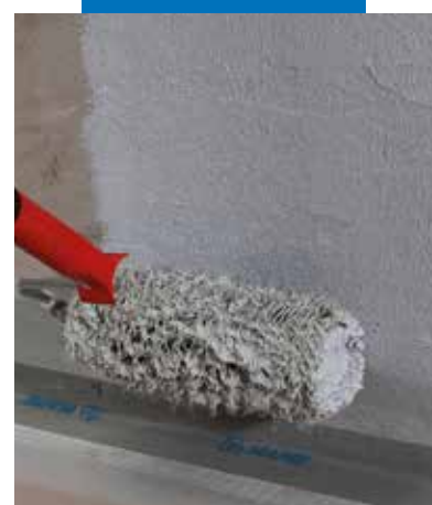
Application of Mapegum WPS with a roller
